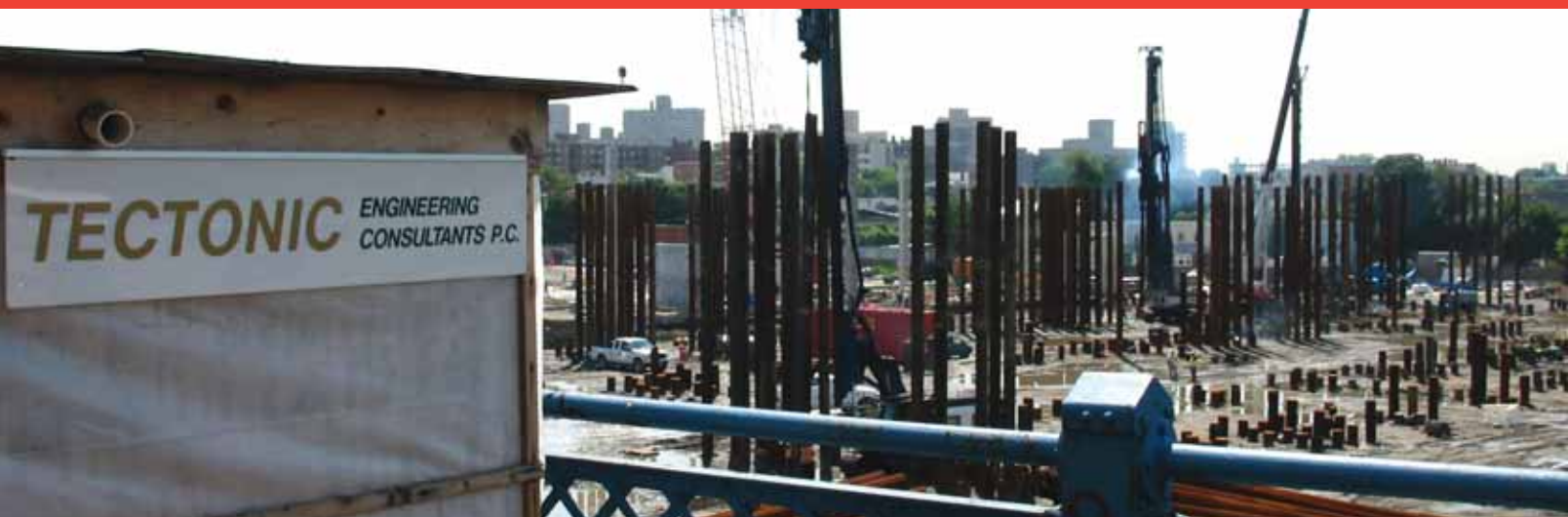
▲ Subway officials feared driving steel piles might cause track movement
